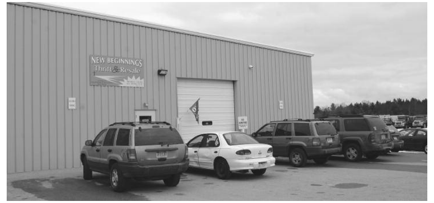
Located at 650 W. Conway Road in Harbor Springs, New Beginnings Thrift Store has an incredible selection of top quality gently used clothing and accessories, furniture, books, jewelry, tons of household items, and much more on display at their 12,000 square foot facility. PHOTO BY DAVE BARAGREY SR.
